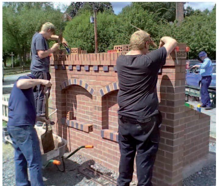
Building the Bunker
